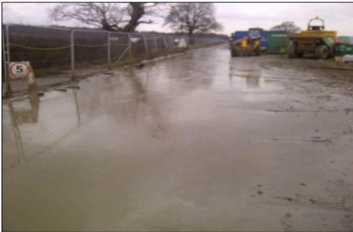
Condition Mid construction
